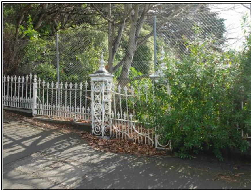
Figure 32 The gateway to the caretaker's cottage on High Street in 2016.
