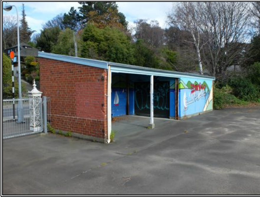
Figure 27 The 1924 boys' shelter shed on the High Street boundary in 2016.
