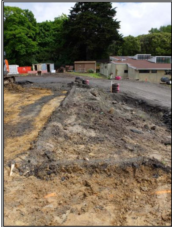
Figure 38 The foundations of the school hall, 29 October 2018.
