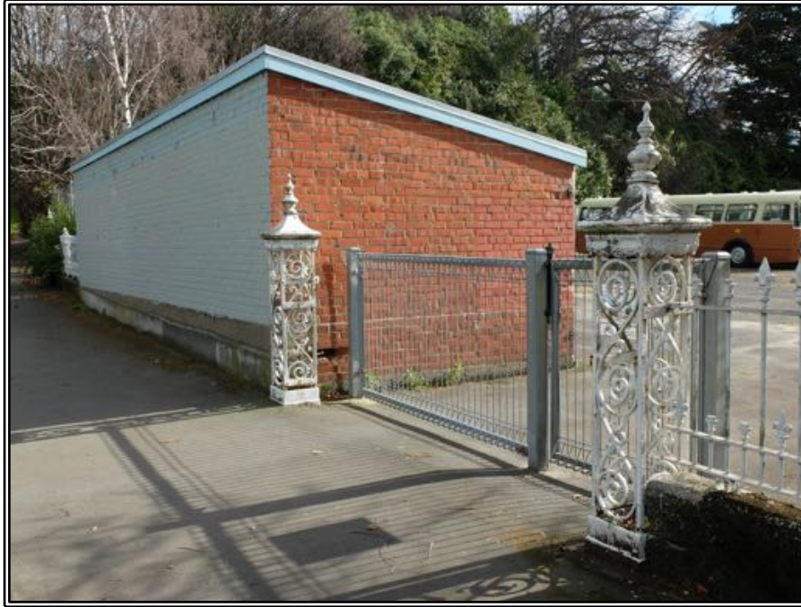
Figure 31 The double gate beside the boys' shelter shed in 2016. This used the 1904 Wrought iron gateposts, but was possibly widened in 1955 to allow coal trucks to enter the school grounds when a new boiler was installed.
