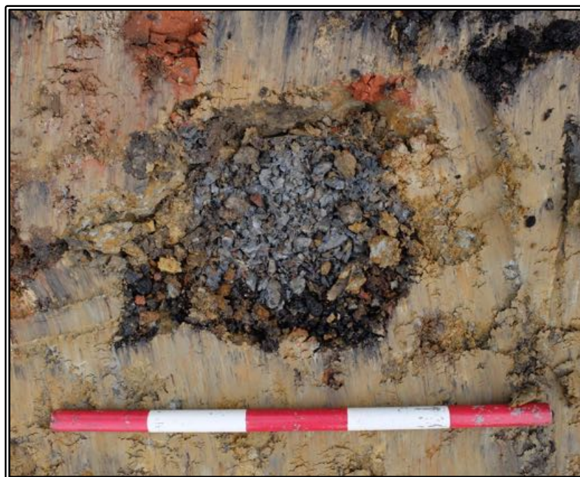
Figure 42 Concrete pile for the caretaker's cottage.
